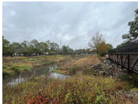
Existing pedestrian bridge along Montilmar Creek Fitness Trail
