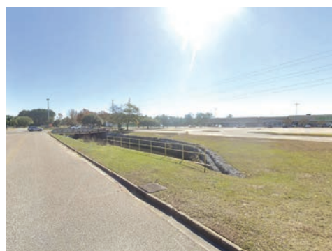
Channelized portion of Eslava Creek
