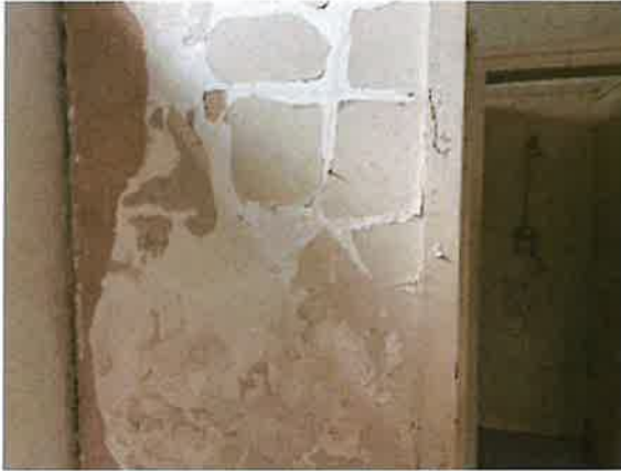
Photo 7 HA-01, wallboard system
