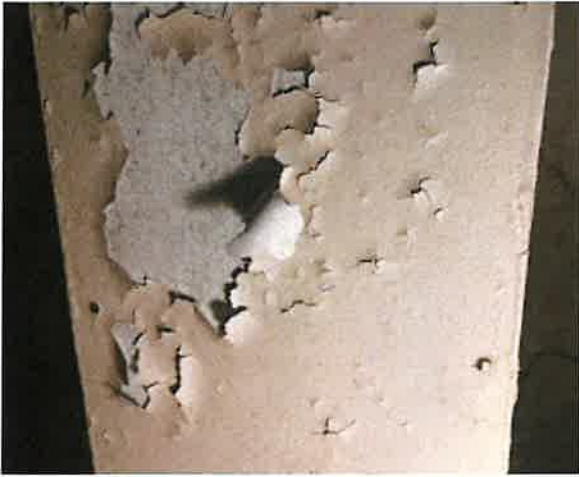
Photo 1 LCP, stage area wall paint
