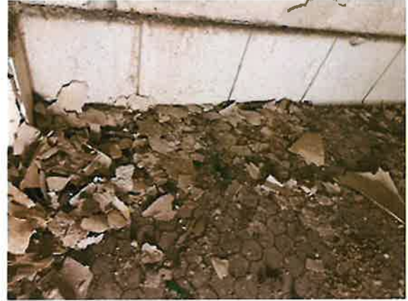
Photo 8 HA-02, baseboard tile
