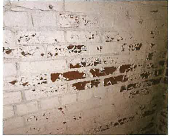
Photo 2 LCP, stage area wall paint
