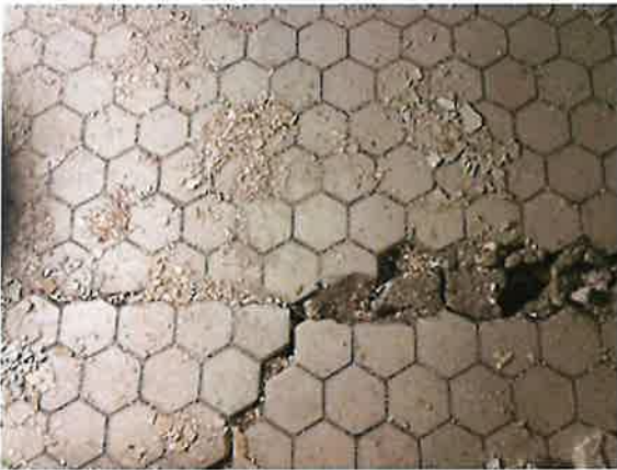
Photo 9 HA-03, floor tile and grout
