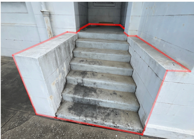
6. Small stairwell with kneewall on right along Water Street
