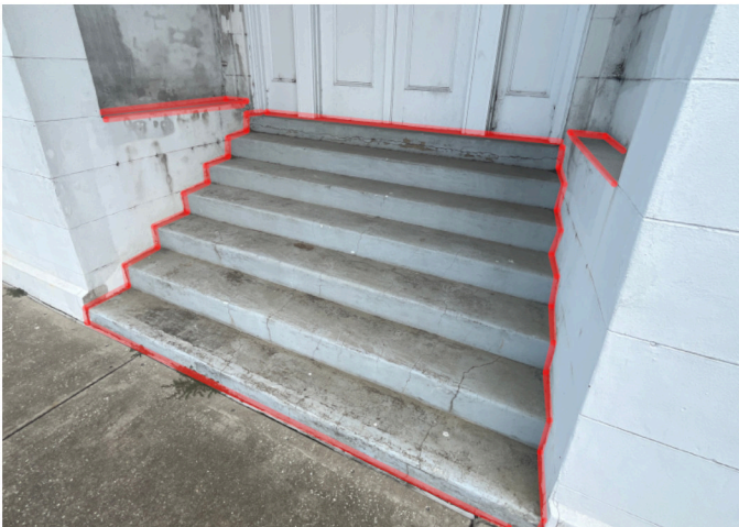
4. Wide Stairwell A along Water Street
