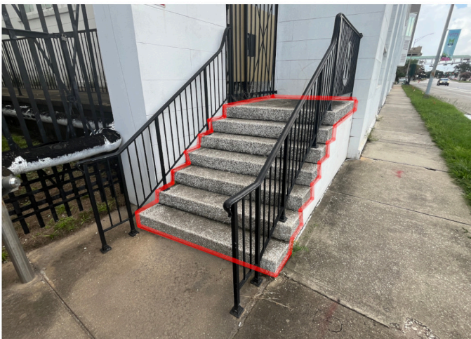
7. Small stairwell with iron railing on right along Water Street
