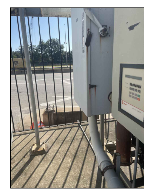
DISCONNECT FOR CHILLER #1 TO BE REMOVED AND REPLACED NEW
